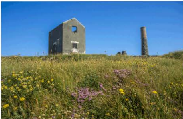
Figure 10.1 Abandoned Copper Mine on the Copper Coast, Waterford County, Ireland
