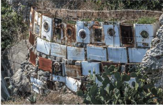
Figure 12.1 Supporting Wall near Matera, Basilicata, Italy
